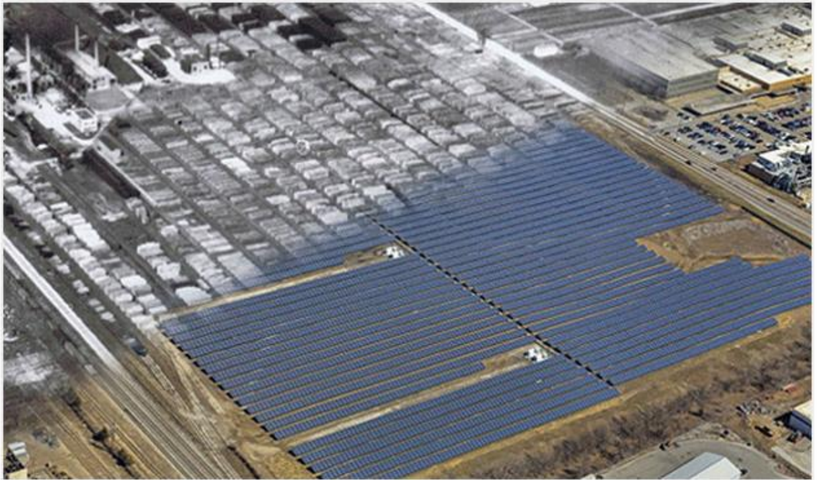
The Reilly Tar & Chemical site in Indianapolis—now home to the Maywood Solar Farm—produced refined chemicals and treated wood products from the 1950s to 1972 (Photo courtesy of Hanwha Q CELLS and Vertellus Specialties, Inc.)
