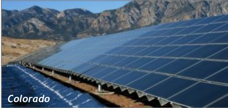
Solar array installed on landfill cap
